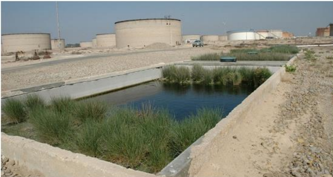
The plants in this Ayala pond treat runoff from the petroleum facility at Kiryat Haim, Israel. Photo: courtesy
