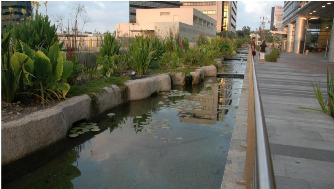
Graywater from a Tel Aviv apartment house is treated for reuse in this Ayala landscape element on the grounds. Photo: courtesy
